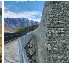
Photo 18 - Bridge approach ramp with steep mesh face MSE wall
