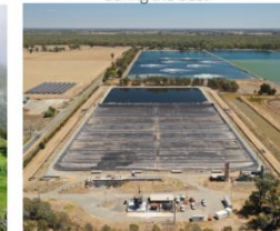
Photo 27 - New HDPE cover on a High rate Anaerobic Lagoon during installation
