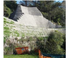
Photo 17 - Shallow landslide protection with reinforced soil embankment
