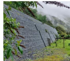
Photo 16 - Slip repair with mesh facing geogrid reinforced soil structure
